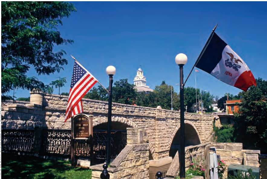
The 1889 Keystone Bridge, Elkader, Iowa
